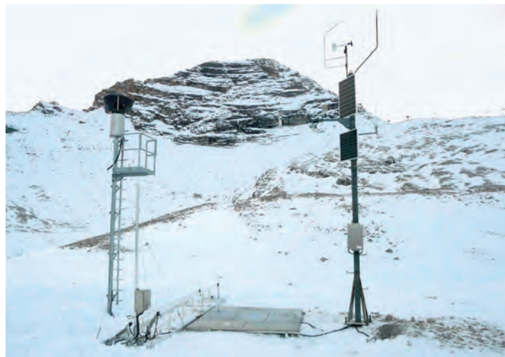
Fig. 8: Meteorological station at central Zugspitzplatt (2420 m a.s.l.), operated by the Bavarian Avalanche Warning Service and the authors on behalf of the Environmental Research Station Schneefernerhaus. It is equipped with sensors for the determination of standard meteorological and snow parameters. The measurement data is recorded and transferred to the Alpine Environmental Data Analysis Center (AlpEnDAC, www.alpendac.eu ), where it is publicly available (Photo: F. Bernauer, 2012-11-08).
